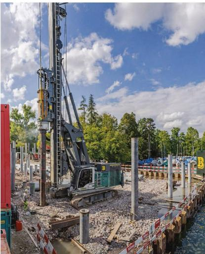
pile driving. Various carrier machines from LRH 100 to LRH 600, but also the complete LRB series are available. Due to the special leader kinematics, very large radii and continuous inclinations can be achieved. Liebherr also has the right tools at the ready with various sizes of hydraulic hammer.
